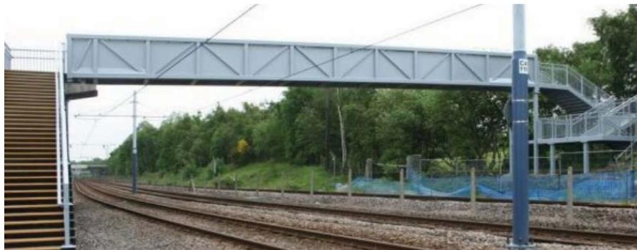
**Photo 5 – Typical half-through footbridge with solid parapets (photo from CTS Bridges)**
